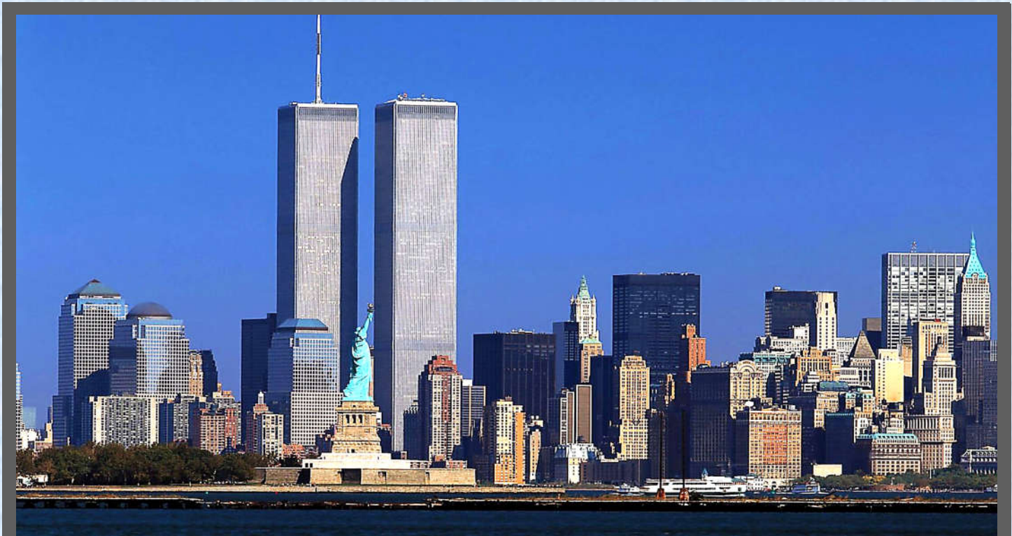
Twin Towers of the World Trade Center (CCASA)
